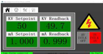
Main Control Screen
